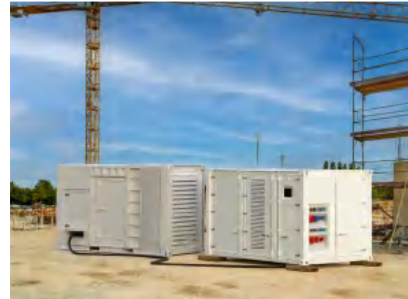
Tower crane Rated power: 45kW Peak Power: 133kW Operation: 10h/day with 2h @100% load, 1h @ 75% load, 2h @ 50% load, 3h @ 25%, 2h @0% load.
